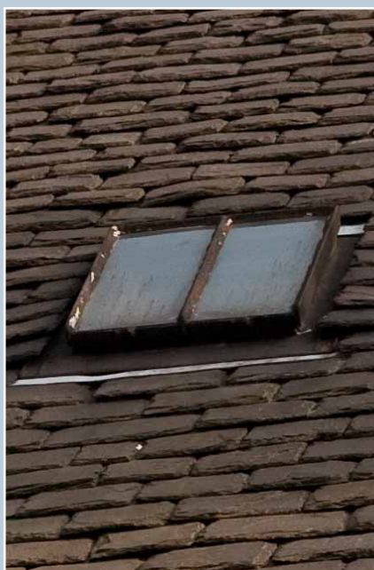
A traditional iron rooflight set into a West Highland slate roof. The small size, low profile and 'portrait' format are typical characteristics. © N. Haynes.
