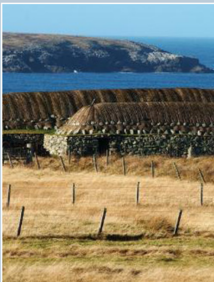
Blackhouse at Arnol, Lewis. Thatching weighted down with stones on ropes.
