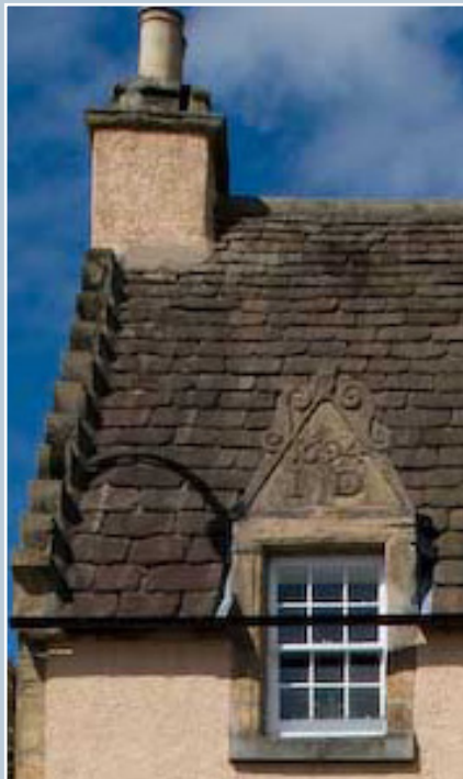
Graded stone slates, laid in diminishing courses from the bottom to the top of the roof. Associated features include crowstepped gables, a corniced chimney and a decorative dormerhead dated 1694. Elgin, Moray. © N. Haynes.
